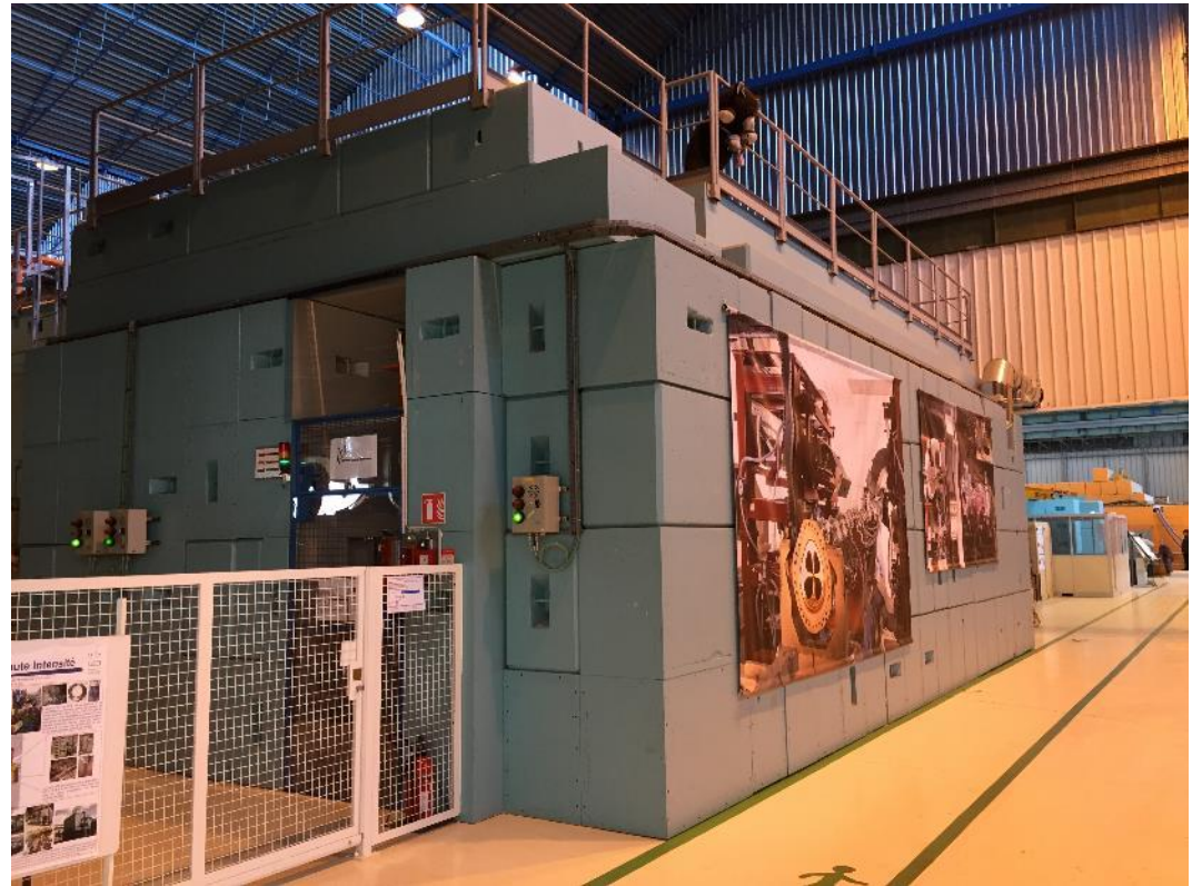
The IPHI Vault @ Saclay
