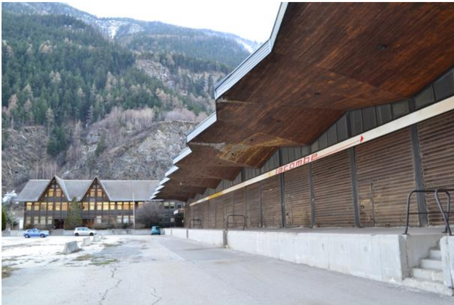
Rented storage for the shielding
