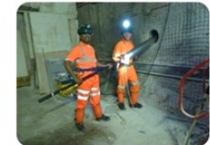
Bore hole detector installation
