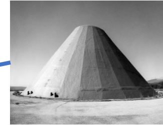
Surface antenna on the top of the mountain (1.016 mast)
