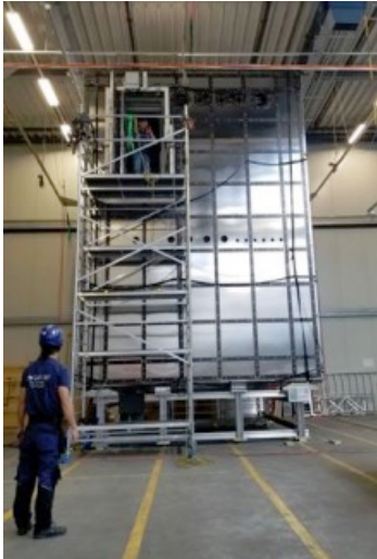
Completed magnetic shielded room at Imedco: Hägendorf, CH
