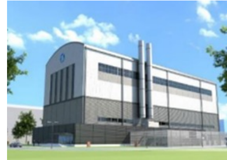
KP-FHR (USA) •320 MWt, 140 MWe design •Hermes demo ORNL (operational in 2027) , Construction permit for the Hermes 2 test plant(2 X 28- MWt)
