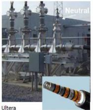
13.2 kV, 3 kA, 200 m Triaxial™ Design BSCCO 2223 Energized 2006 High reliability 1
